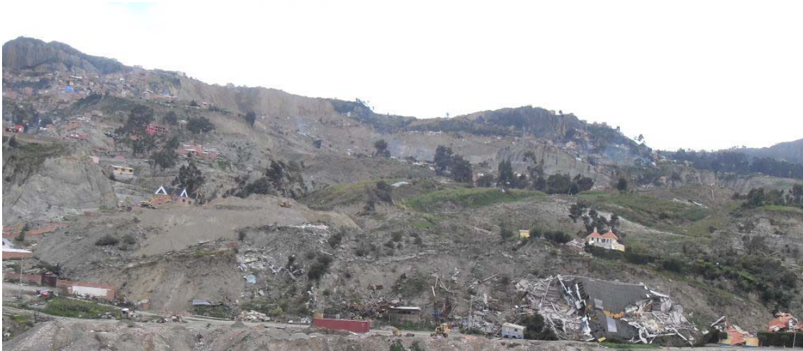
Fig 1.c Area of mudslide along the side of the mountain downhill.
